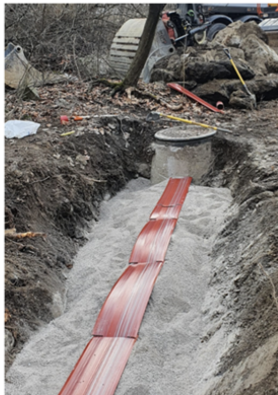
Figur 13d: Kabelmarkering.
