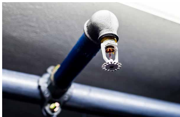
You must never disconnect or hang anything from sprinkler heads.
