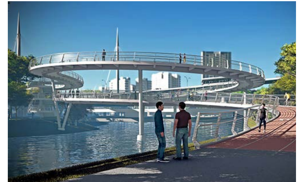
Spiral bridge, Pier 1 (Kilde: todayonline.com)
