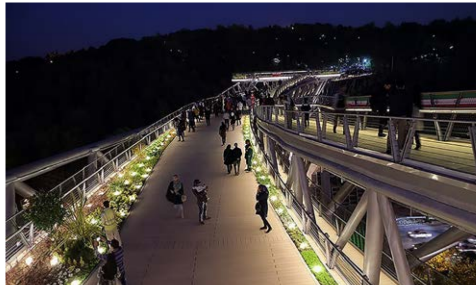
Iran's largest Pedestrian Bridge called "Tabiat Bridge" (Nature Bridge) in Tehran. (Kilde: realiran.org)
